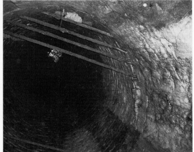
Remains of steel guard bars in Highclere Shaft.
